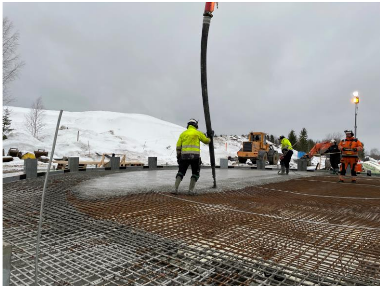
Gjutning 90 Kbm betong, RK1
