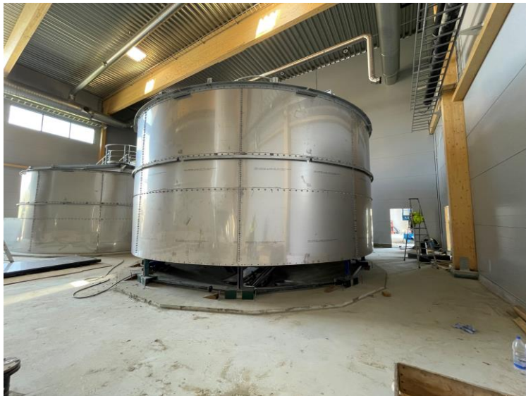
Tankmontage i processhall
